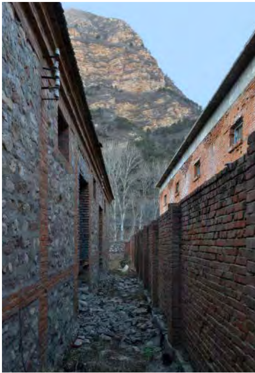
Escapist Resort Site Condition
