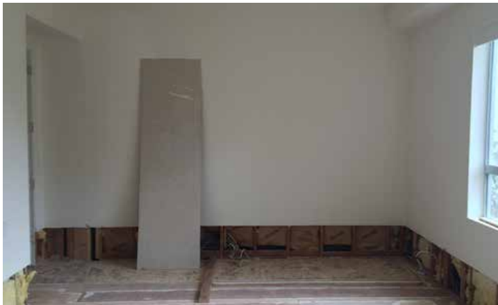
Guestroom: Existing Condition
